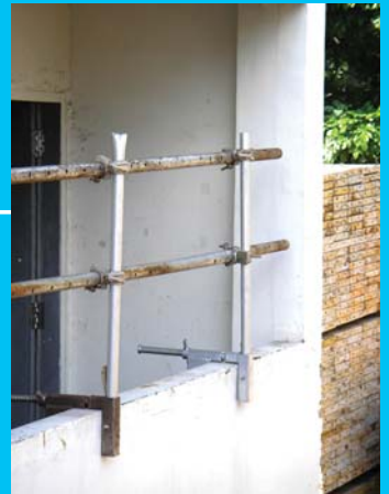
EP + Tubes & Fittings On Upstand beams
