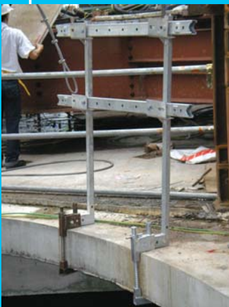
EP + Railing Post + Guardrails (S) On Slab
