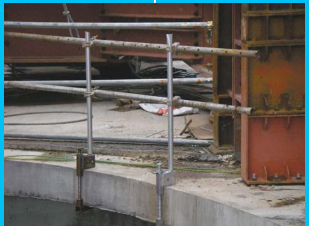
EP + Tubes & Fittings On Slab
